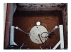
SBR and Digester decanting pump is equipped with a suspended solids sensor that allows the decanter pump to operate independently. When the suspended solids rise above the set value, the sensor will activate shutting down the decanter, ensuring that only supernatant water is discharged without any entrapment of sediment.
