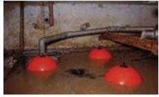
The unique FSP scum skimmer removes floating oils and grease solids. The scum is pumped from the skimmer to the concentration tank for processing.
