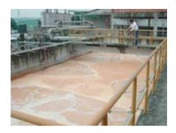
The BER is designed for both very high oxygen transfer and excellent mixing.
