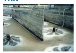
Submersible aspirating aerators ranging in size from 1HP to 55HP. The TRN provides very high oxygen transfer efficiency and mixing.
